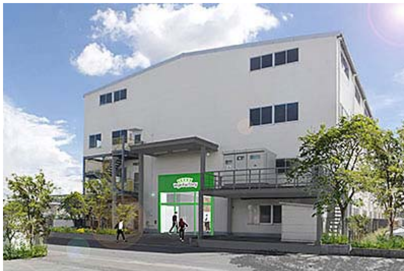
Sugito Factory to Demonstrate Mass Production scheduled to be completed in July 2021
