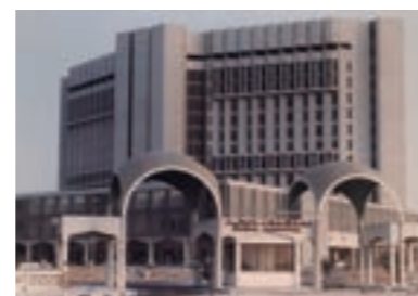
New Dubai Hospital
