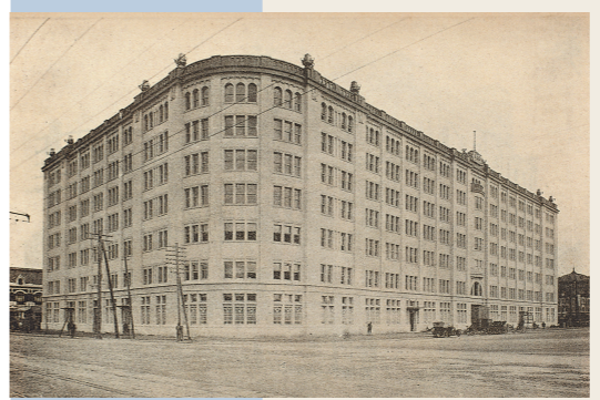
Tokio Marine and Fire Insurance Building
