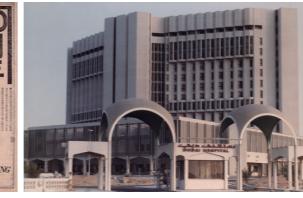
1981 Air-conditioning, water supply and drainage, hygiene, electrical and medical-use gas supply facility works for New Dubai Hospital (United Arab Emirates)
