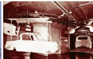
1961 Drying Oven for the R360 Coupe at the Toyo Kogyo Co., Ltd. F Plant
