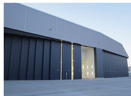
Appearance of the paint finishing plant Photo courtesy of MHI Plant Engineering & Construction Co., Ltd.
