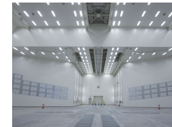
Inside the paint finishing plant Booth B
