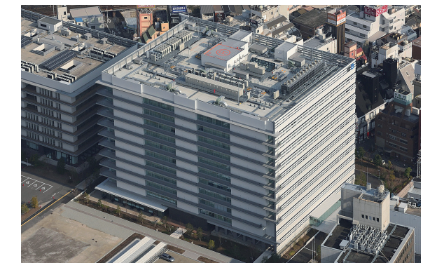
NTT West Training Center Shinkyobashi Building
