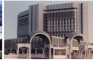
1981 Air-conditioning, water supply and drainage, hygiene, electrical and medical-use gas supply facility works for New Dubai Hospital (United Arab Emirates)
