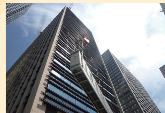
Load-lifting work for condensing unit
